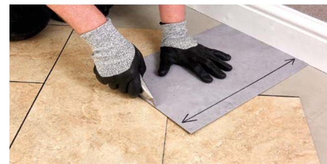
Figure 9 Cutting the perimeter tiles (diagonal cut)
