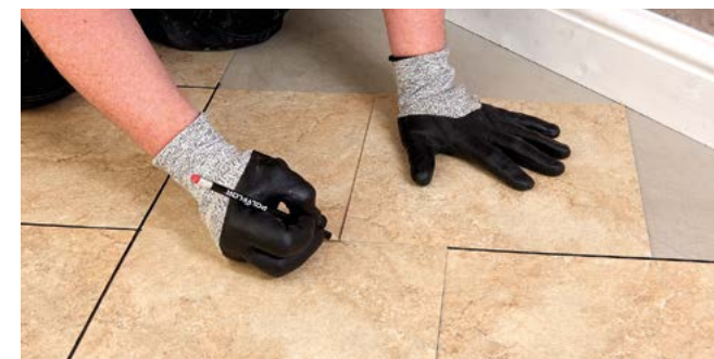
Figure 8 Marking using an overlapping template on diagonal laid tiles
