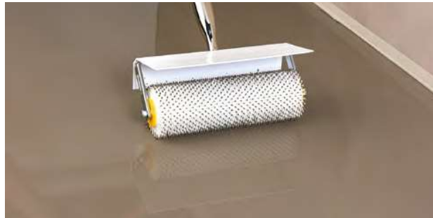
Figure 2.1 Spiked screed roller
